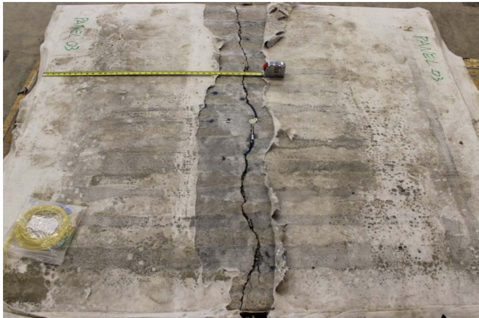
Fig. 6.8. Cracks in P3 after load frame test.
